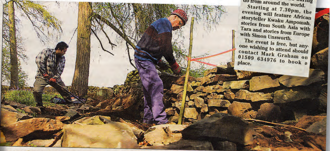
CONCENTRATION: Conservation volunteers are busy restoring dry-stone walls at The Outwoods, near Nanpantan
