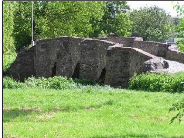
Packhorse Bridge over Rothley Brook
