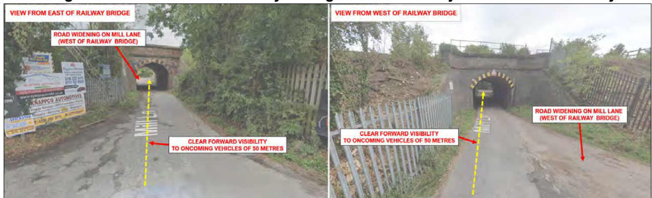
Figure 4A Forward Visibility along Mill Lane adjacent to Fosse Way
