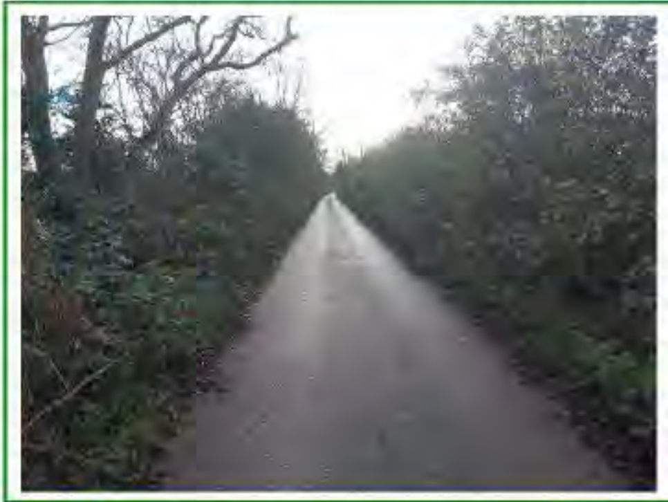
Photo No.4: Facing SE from the entrance to the main site area showing the continuation of Mill Lane / site access route
