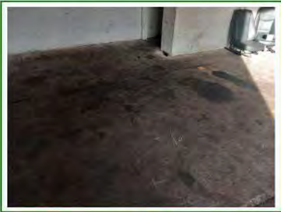
Photo No.31: Interior of Unit No. 17 A/B/C showing oil staining throughout (olfactory evidence of hydrocarbon presence noted)
