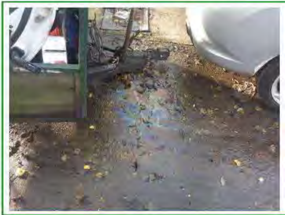
Photo No.76: Iridescence noted atop concrete adj. to trailer containing chemicals / fuels etc in car-parking area in north of site
