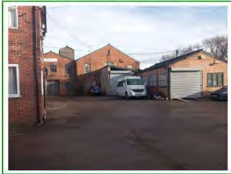
Photo No.66: Facing east / NE from the car-parking area in the north of site towards Units No.18 and rear of Unit No.17 A/B/C
