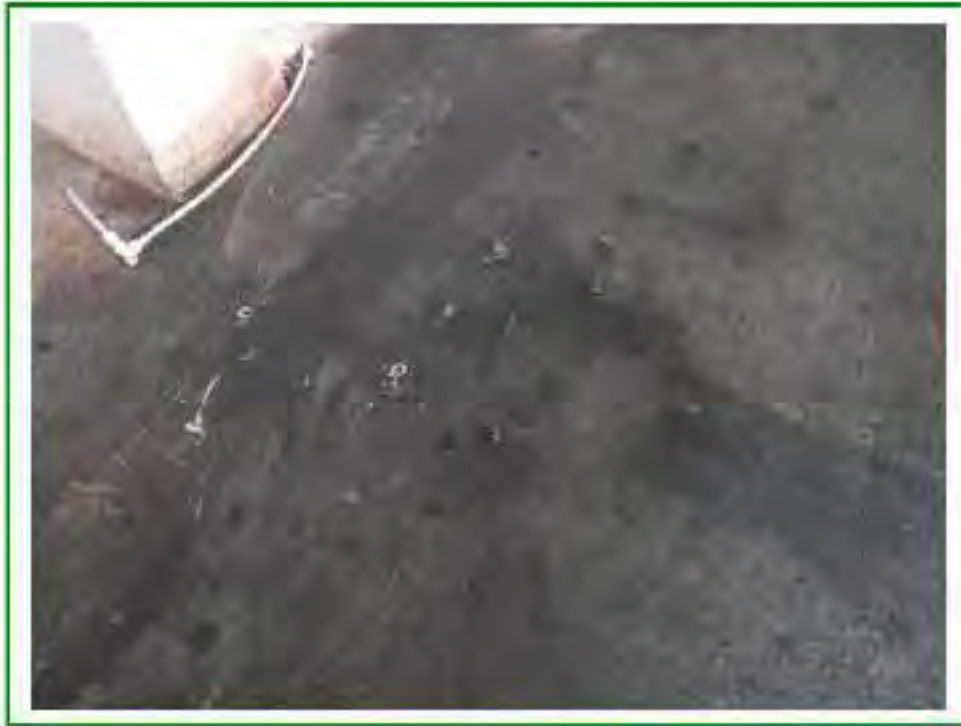
Photo No.32: Interior of Unit No. 17 A/B/C showing oil staining throughout and former vehicle lift location (bolts)
