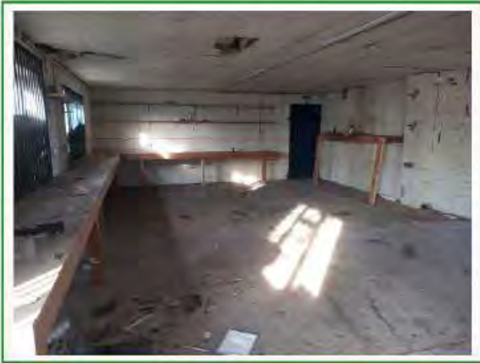
Photo No.62: Showing interior of Unit No.7/7A (rear room)
