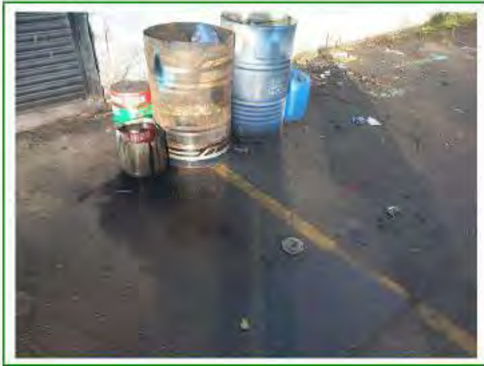
Photo No.64: Further open-air, uncovered barrel / oil & hydrocarbon storage with evident release noted
