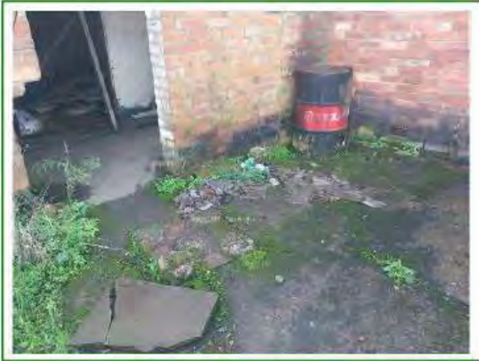
Photo No.38: Showing area between Units No.10 (O) and 16 with further oil / barrel and fragmented PACM storage noted
