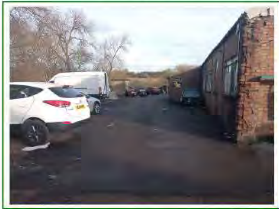
Photo No.46: Facing NE in the far west of site showing the rear of Units A, C and B1/B2 (river to left of photograph)
