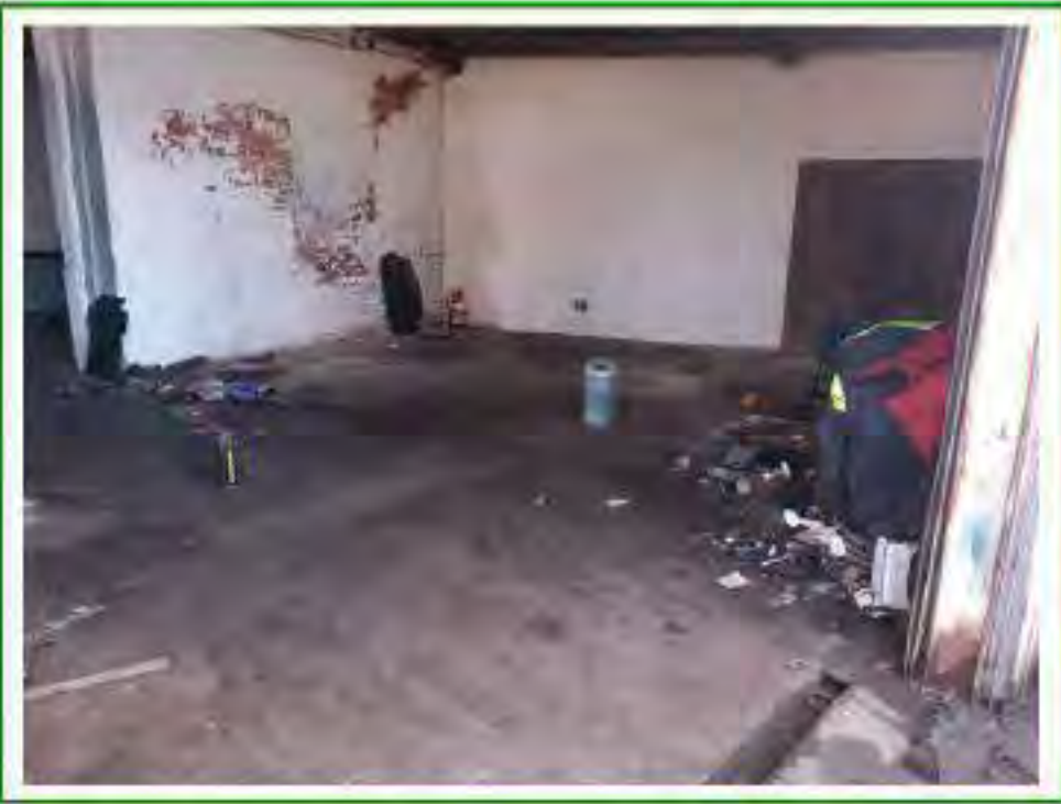
Photo No.69: Interior of Unit No.16 showing scattered debris and significant hydrocarbon staining on flooring
