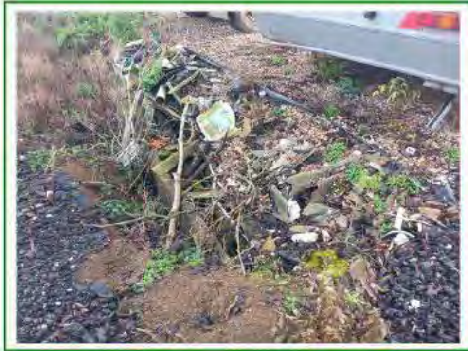
Photo No.22: Former wall located between Plots No.105& 106 showing significant PACM and made ground presence
