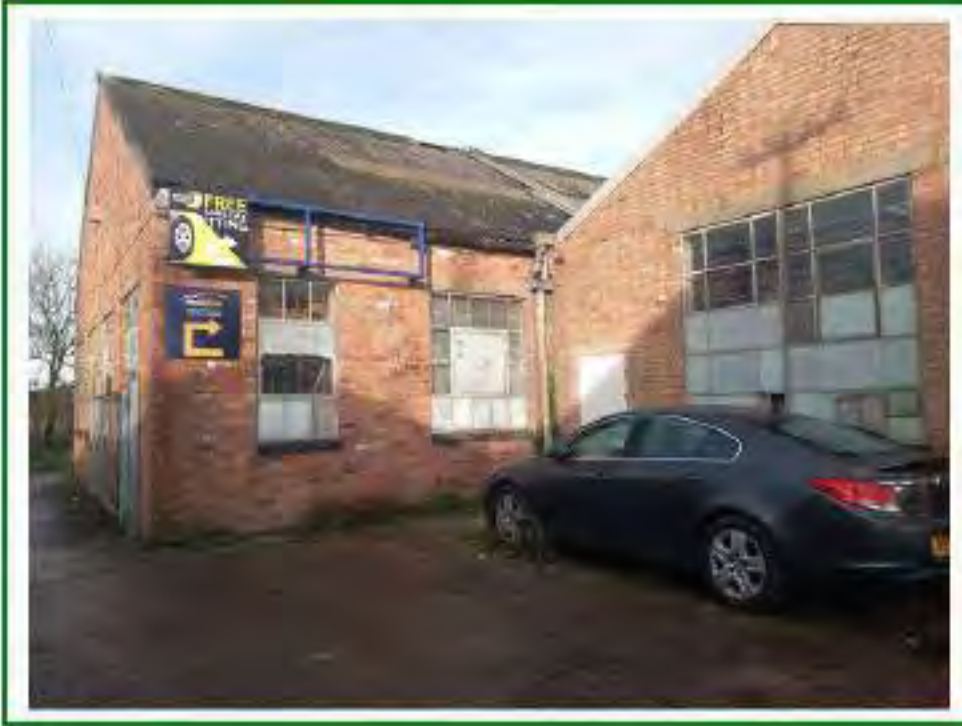
Photo No.58: Facing north showing Units No.B1/B2
