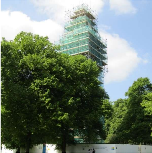
The Carillon clothed in scaffolding during refurbishment work in 2018
