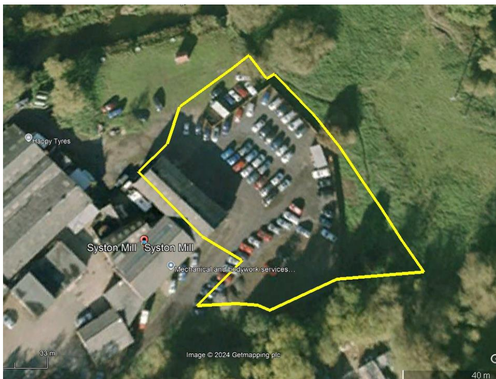
Figure 10 - Aerial photograph from 01 January 2010 with approximate area E-Lease now occupy outlined in yellow.
